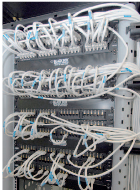
The AMPTRAC patch panels enable the patch status of each individual port to be traced.
