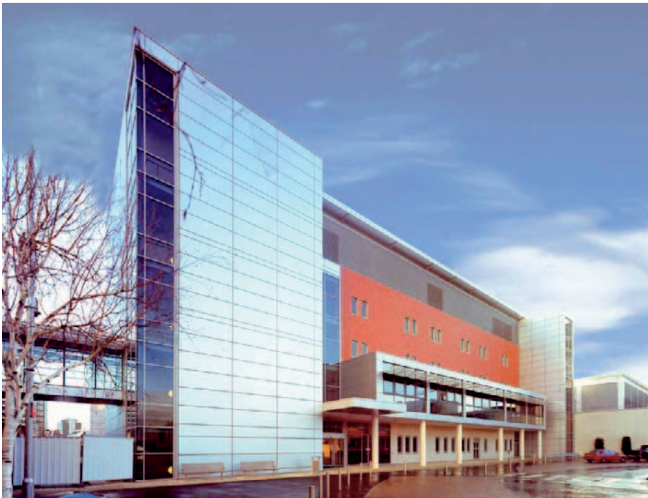
The Cancer Centre of Belfast City Hospital is a modern, attractive state of the art building. It hosts the radiology suite, research facilities and also 84 inpatient beds.
